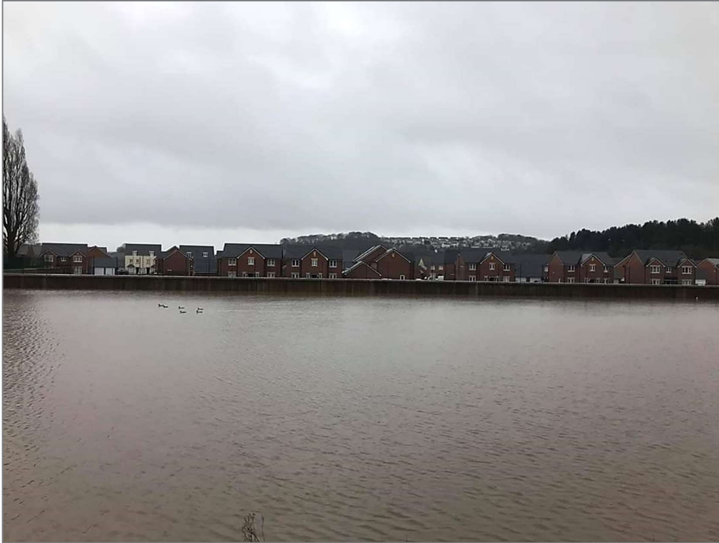
FIGURE 14: FLOOD DEFENCES AT JUBILEE PARK (H1(54)) FOLLOWING STORM DENNIS IN FEBRUARY 2020
